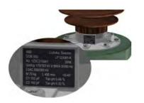
Capacity C1 and tan $\delta$  / PF under factory testing are documented on name plate of bushing
